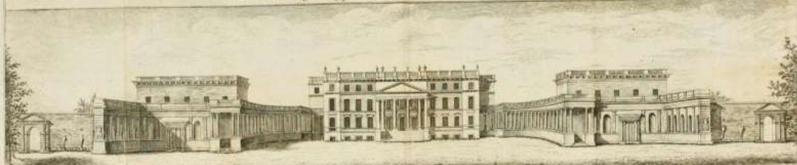
The North-West Prospect, or Park Front of Stowe House.
